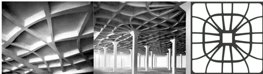
Figure 3 a,b,c: Nervi's work demonstrates a strong correlation between aesthetics, statics, materials and construction technology. This is evidenced in the mezzanine slab in the Palazzo dello Sport and the Gatti Wool factory. These have been studied to gain tangible insight into Nervi's intuition and working method.
