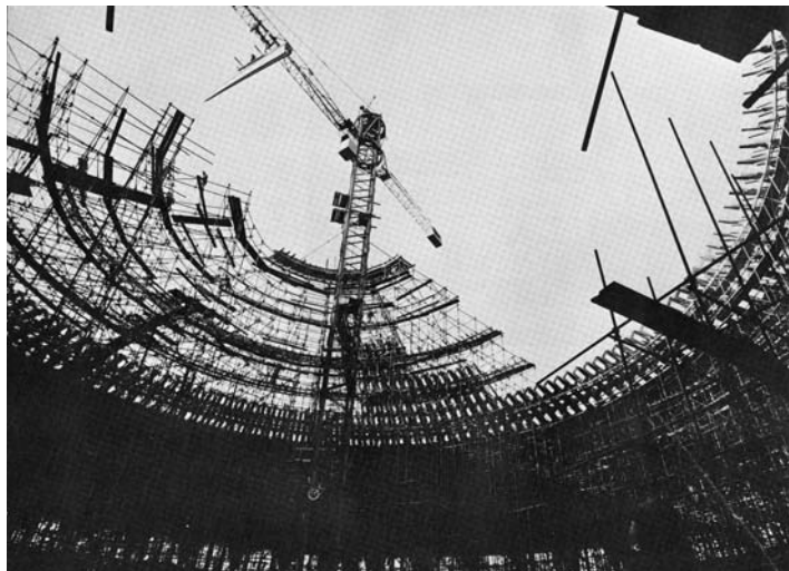
Figure 7: Construction photo of the Palazzo dello Sport, Rome. An array of precast elements form the dome.
